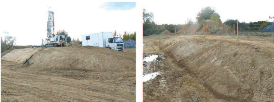
Figure 7. View of the experimental dry dikes built at the Rouen Experimentation and Research Center: on left the lime treated dike and on right the untreated dike.
